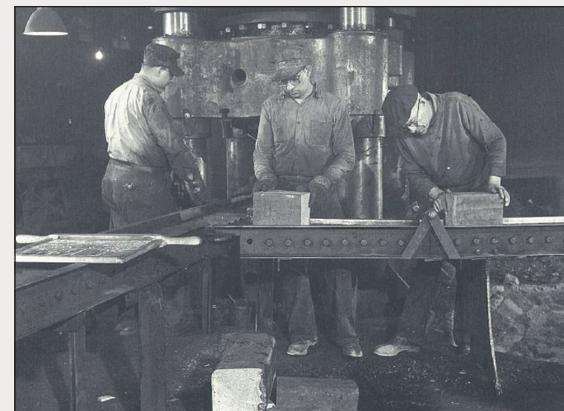
Steel Billets for Cylinder Manufacture
