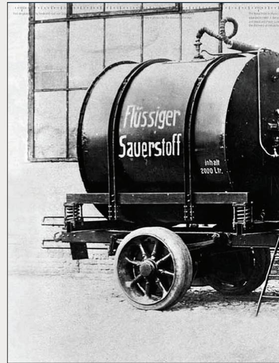
First Portable Tank for Liquid Oxygen
