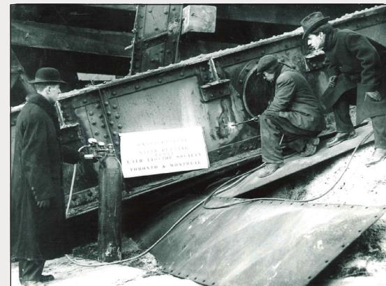
1915 Oxy-Acetylene Welding Demonstration
